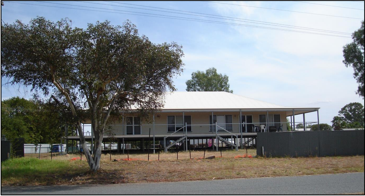
Above: The site in March 2019. The old hotel building has been demolished and replaced with a totally new structure.
