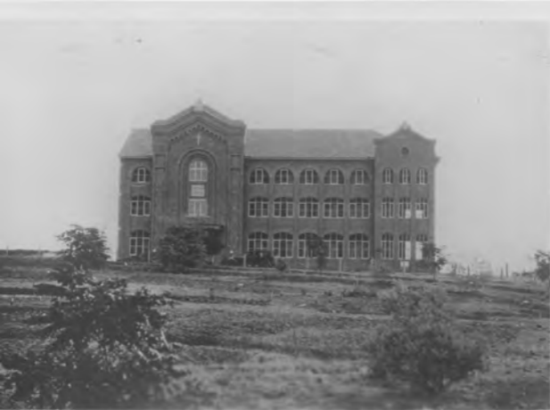
LEWISHAM HOSPITAL. WAGGA, N.S.W.
