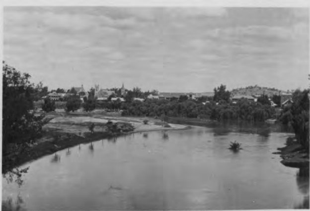
VIEW FROM HAMPDEN BRIDGE, WAGGA
